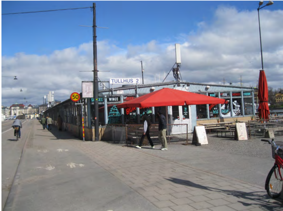
Figure 5: The figure shows base stations on a one floor building, Tullhus 2. Note the low position causing high RF radiation levels to people passing by such as pedestrians and cyclists on Skeppsbron.
